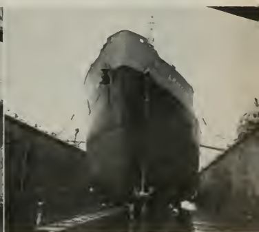
Painters cleaning bottom before application of bottom paint. Man with long marker stick is marking deep load line on the ship's bow.
